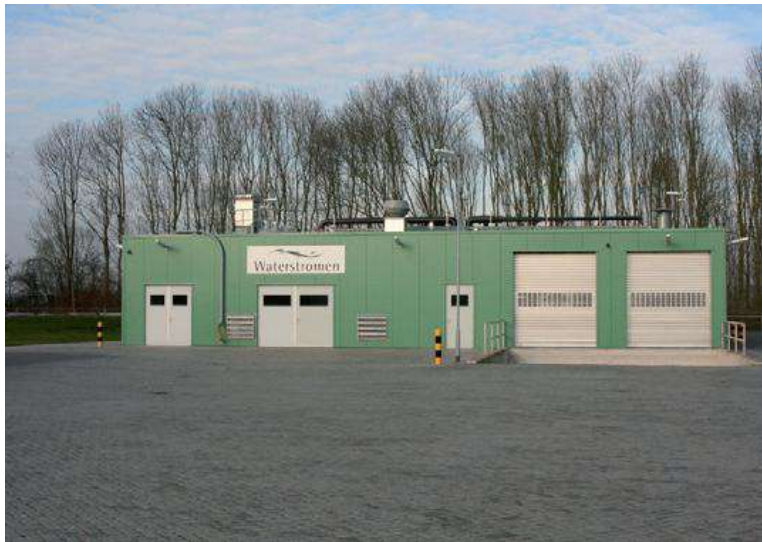
Full scale plant at Olburgen WwTW, Netherlands
